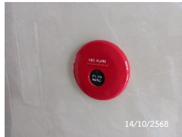
Fire Alarm Manual Station
